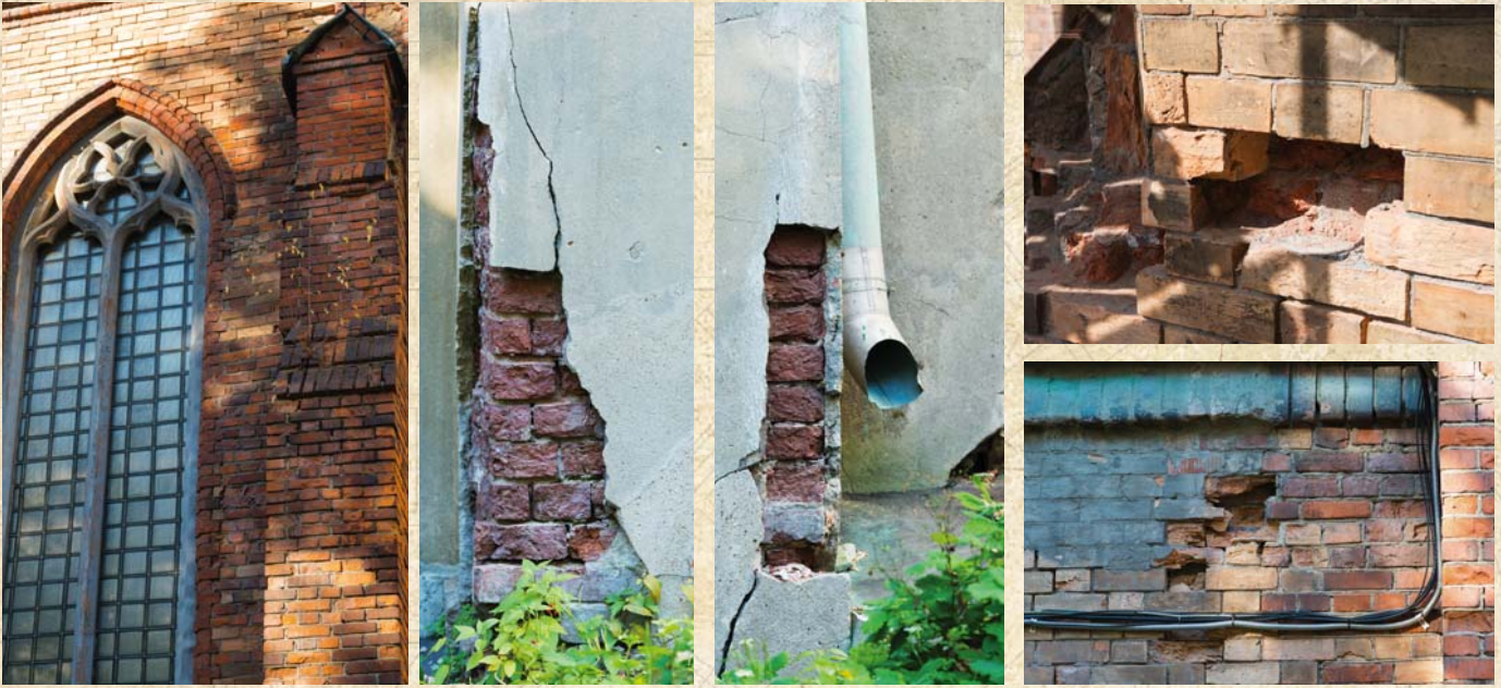
The ravages of time and weather: a 19th Century architectural treasure in urgent need of restoration.
